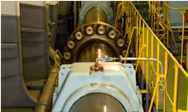
Propeller shaft
